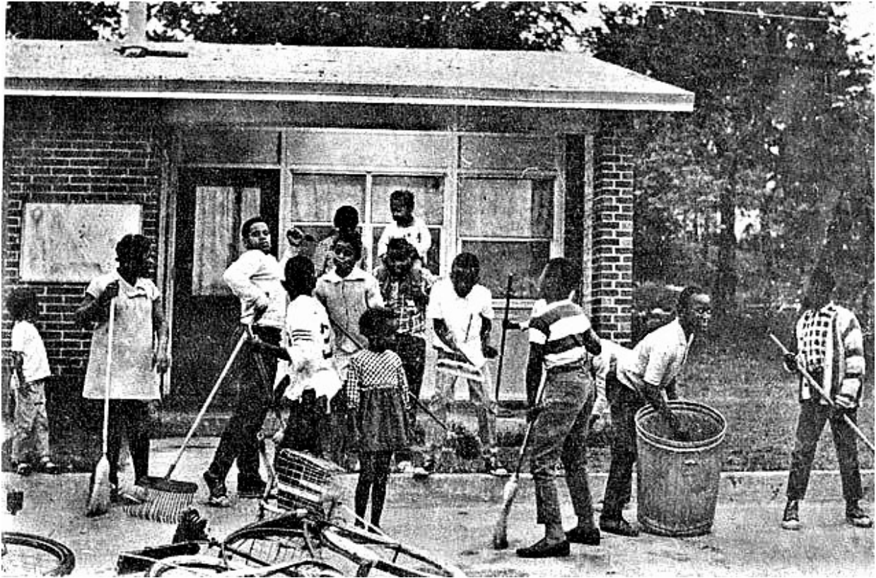
Figure 6-86. Sutterlin Terrace, 1968 Source: Kentucky Historical Society
