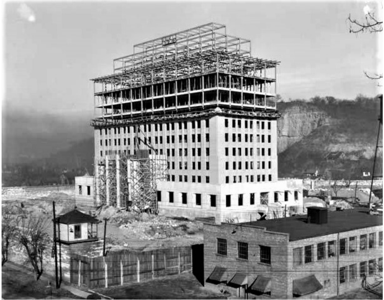
Figure 6-55. State Office Building Under Construction, 1939 Source: Kentucky Historical Society
