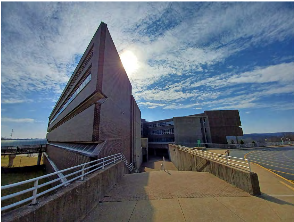
Figure 8-9. J.S. Hathaway Hall at KSU, 2022 Source: Robbie D. Jones
